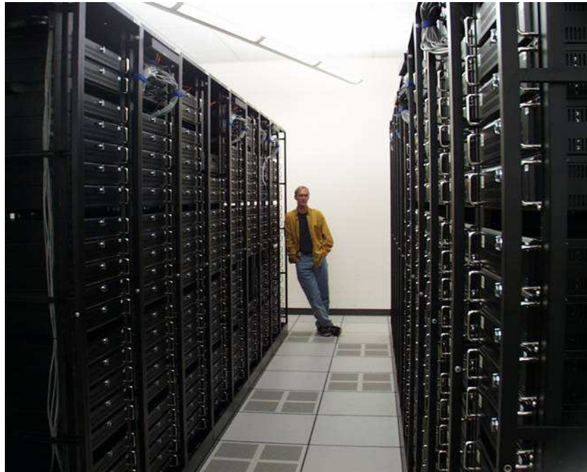
Figure 4. A commercial server farm composed of clustered servers can fill a large room.
